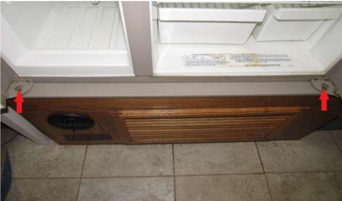
Re-install the rear mounting screws (RA). Refasten your defrost hose
