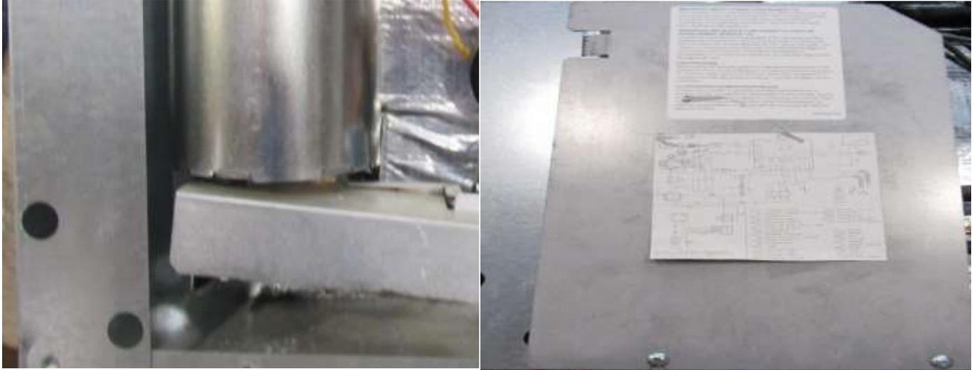
Most times Your fridge has 2 or more vent fans on the center of the unit blowing air up, these can be reattached same as they were on the old unit, make sure they are pointed up and the fan switch needs to be located on the plate marked "fan switch" shown later. Or if you bought our recommended vent fan kit it gets mounted to the back of the unit marked "Fan Backer" this has a thin sheet metal backer to hold the fan into place.
