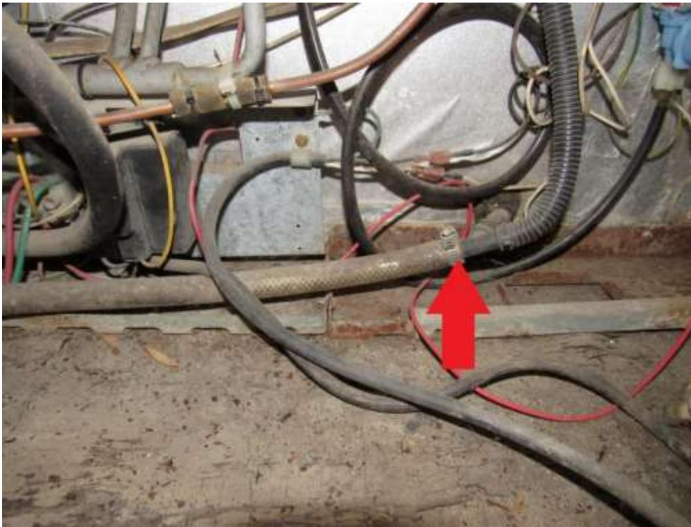
Turn water pump off, remove water supply line from the ice maker valve (RA).
