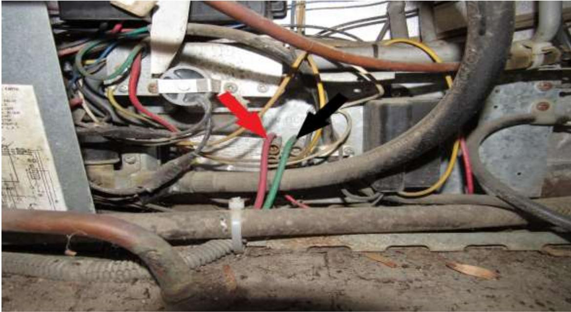
The color of the wires will vary but the 12V positive wire (**RA**) is always on the left and the 12V negative wire is on the right. Wires are not insulated so you will need to put a piece of tape or a twist cap on the 12V positive side (**RA**).
