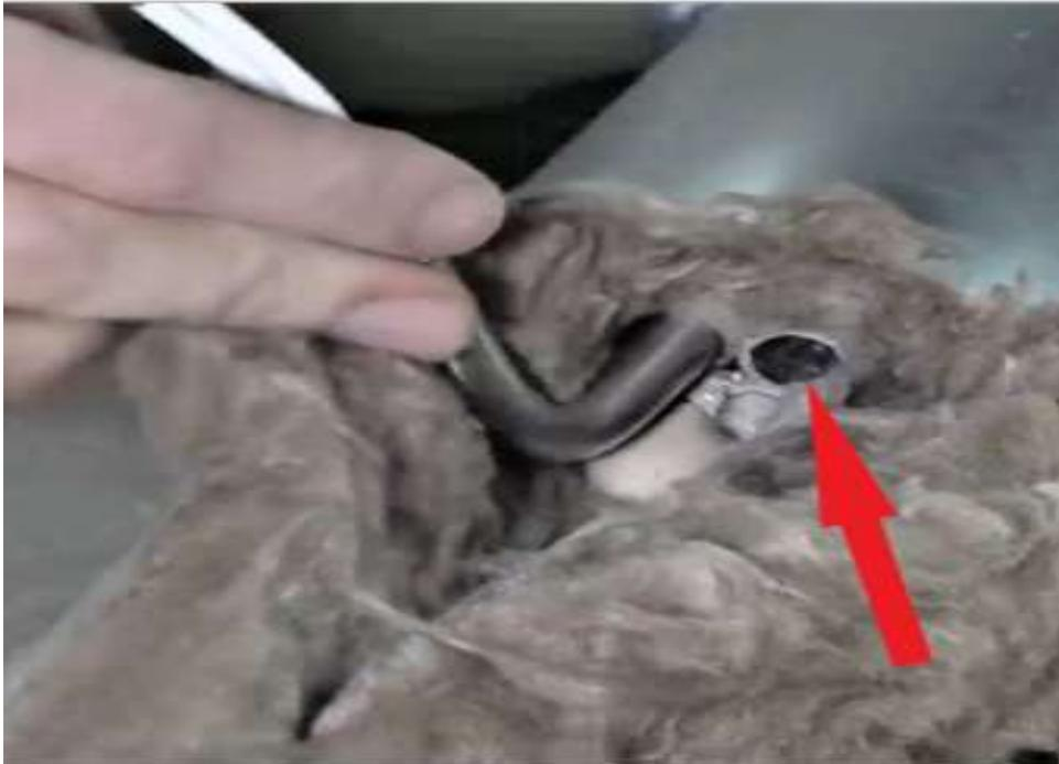
Make sure the heaters are turned towards the inside of the unit so the cover will fit better later (RA)
