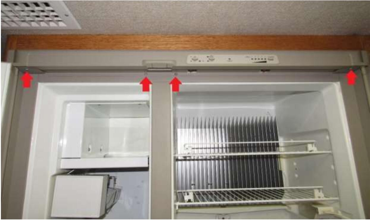
Remove two top mounting screws (**RA**).
