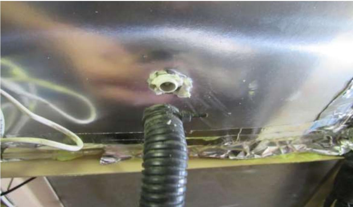
Make sure defrost hose is pushed tight into the cup spigot.
