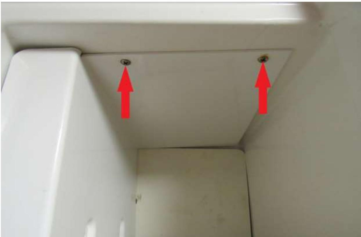
Lay horizontal pc on top and insert the bolts into the bottom freezer plate (YA). Using a small pry bar works very well by inserting it between the freezer sidewall and plate as shown providing pressure against side plate to eliminate gaps (RA). This may need to be pushed or pulled to get it into place.
