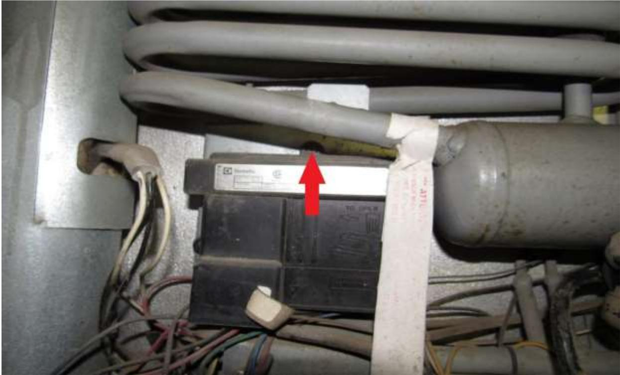
Remove three wire harness plugs (RA) and heating element wires (YA).
