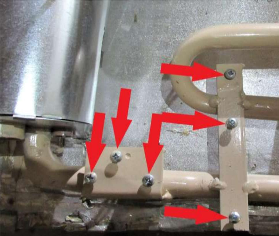
Slide the board/burner housing into place again, same as before
