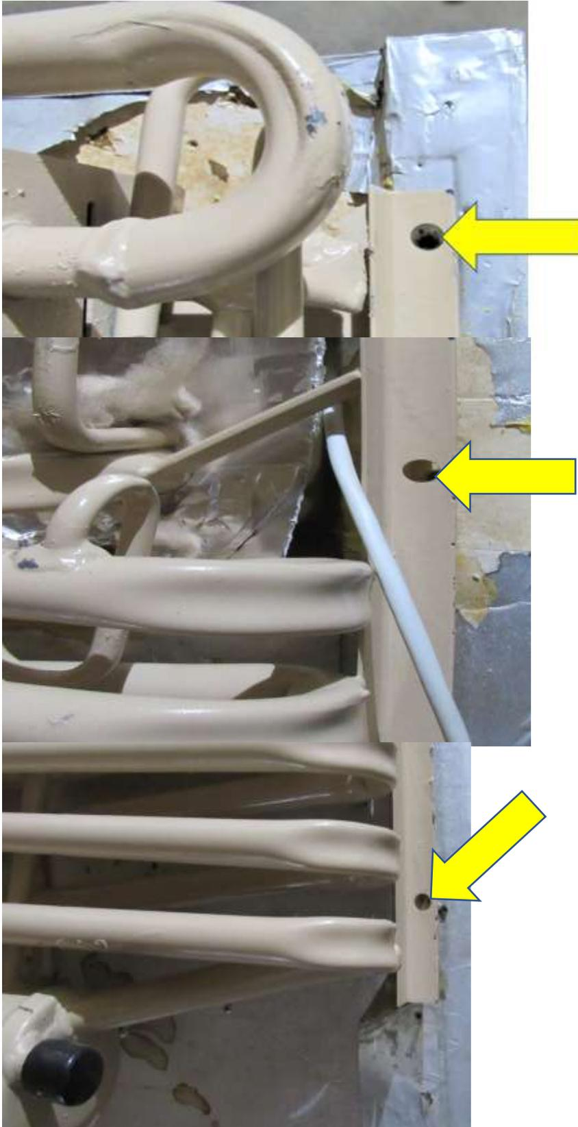
Remove these screws from burner mounting brackets (RA)
