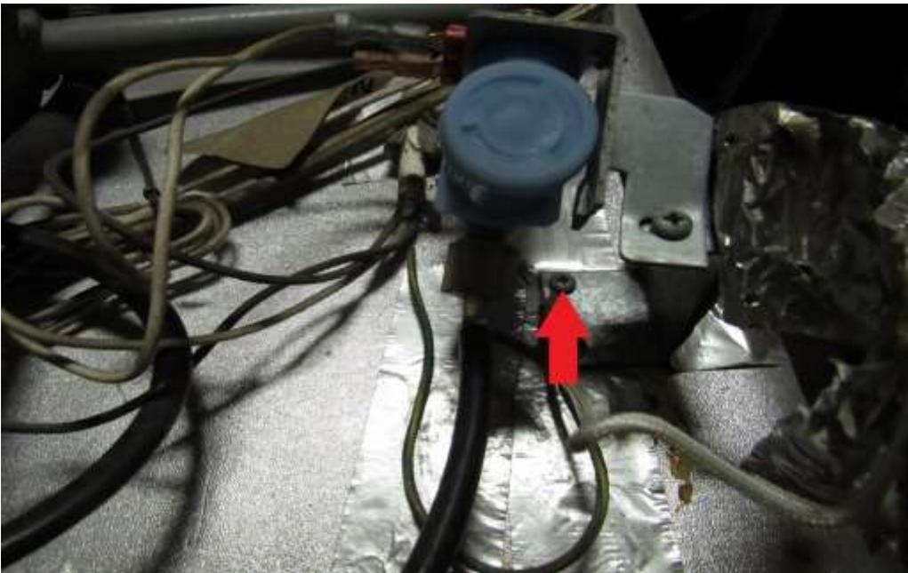
Remove the 120V wires from ice maker cord (RA).
