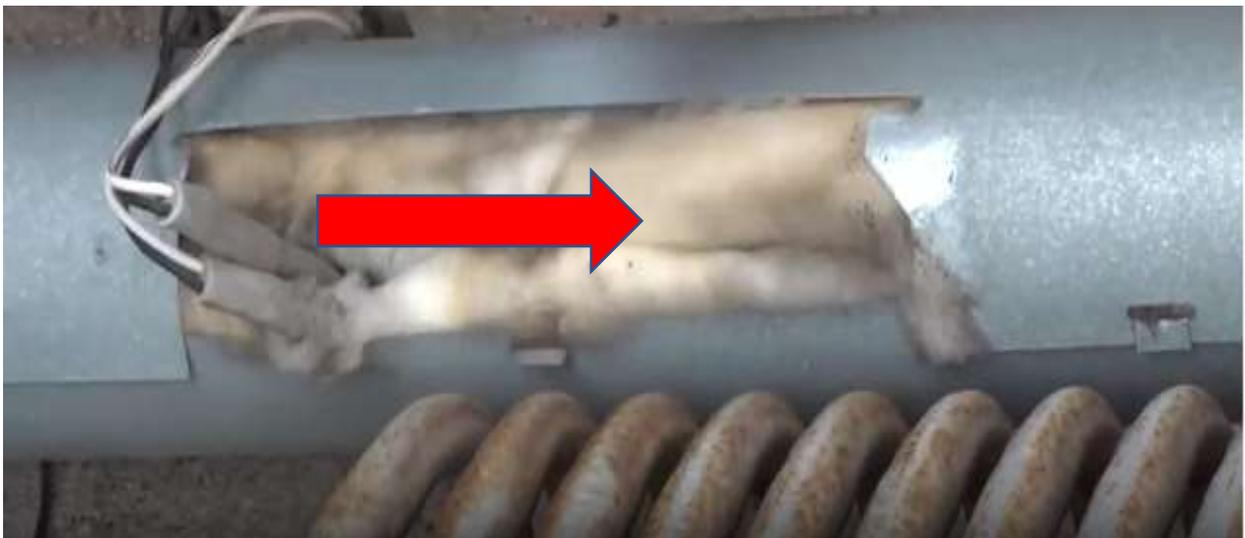
Now lay the new unit on its face carefully and open the heater flapper as well and push insulation to the side to find the 2 sockets (RA) that the heaters will slide into. Make sure heaters are slid in all the way down as far as they go. Tuck the insulation back around the heaters again and close the flapper
