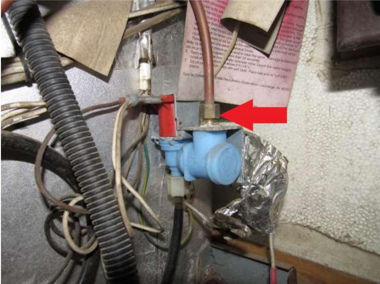
Make sure LP gas is turned off. Remove the LP gas line from the solenoid (RA).
