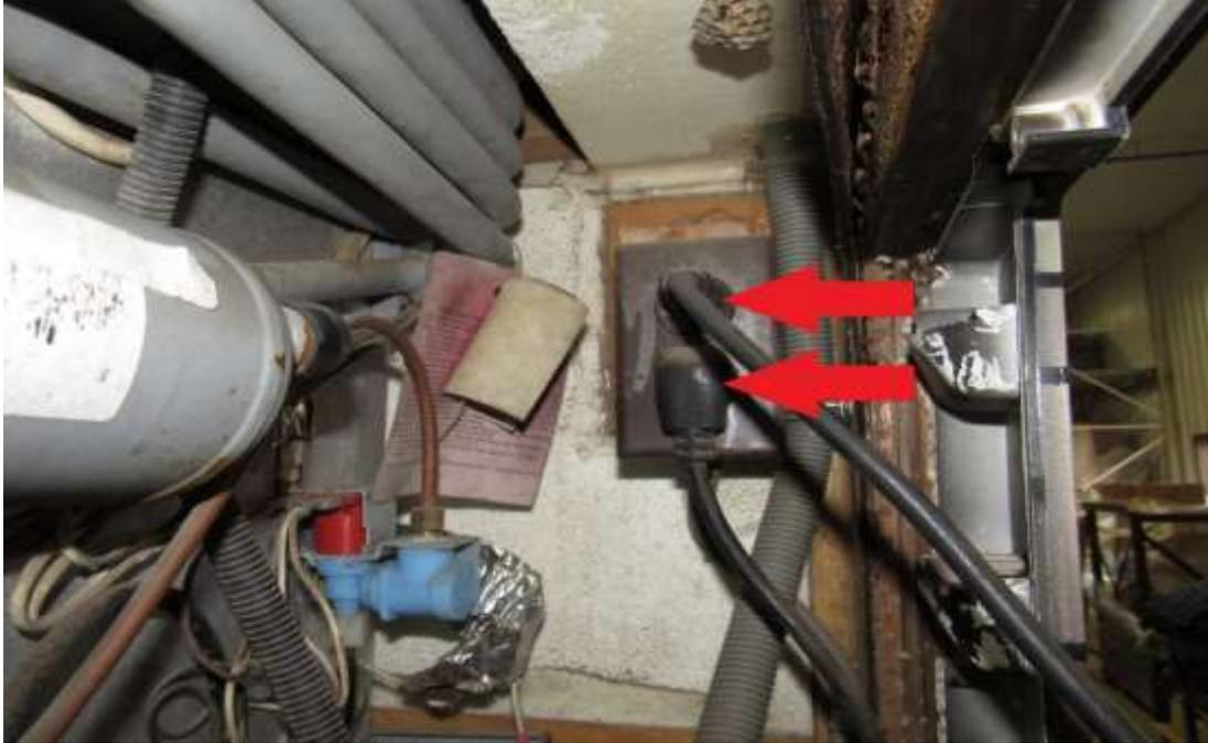
Remove defrost hose from the "T" (RA). Placement could vary.
