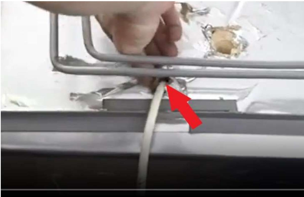
Lift unit straight up and out of box. This can be very tight as some of the older ones are really sealed in tight. Use a pry bar (RA) and a piece of steel (YA) for a backer to break the seal on the unit. If yours has fans you will want to remove these for later, otherwise if no fans are there it will be shown later how to install new ones as these are required on all new units. (GA)
