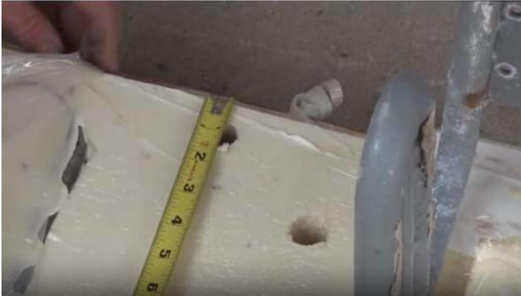
New unit, these should be drilled at a slight angle downward so the water out of the spigot runs into the icemaker.
