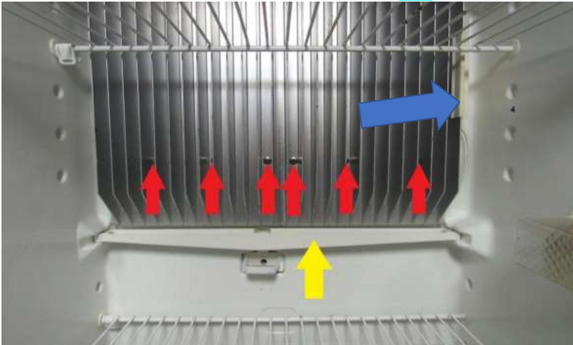
Remove the top plate mounting screws in freezer (RA).
