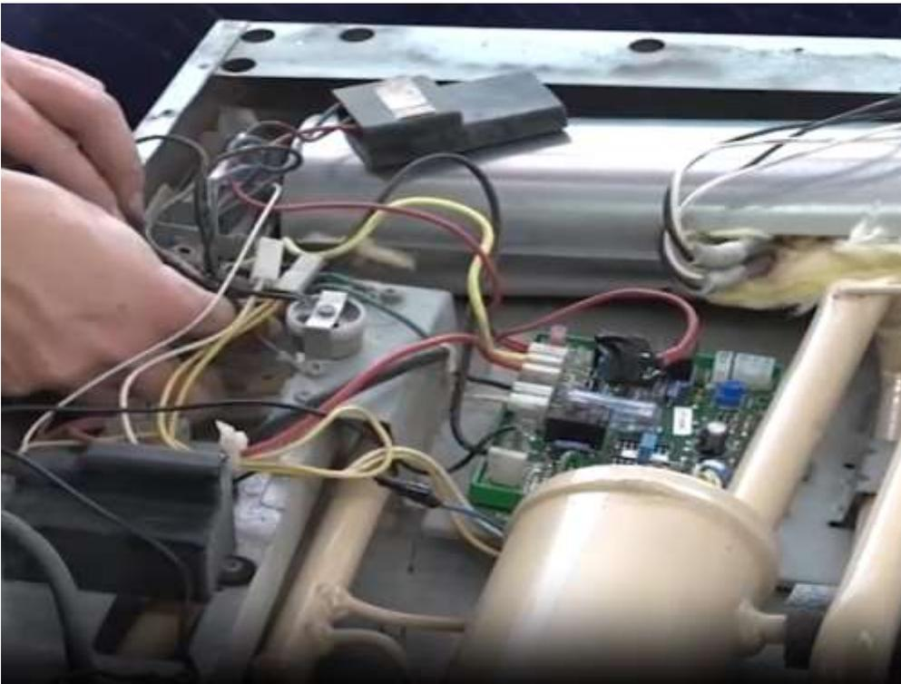
Lay burner back onto bracket, make sure LP Burner is up against the bottom of the flue tube (YA) need approx. 1/8" gap between burner and igniter (GA) Styles may vary
