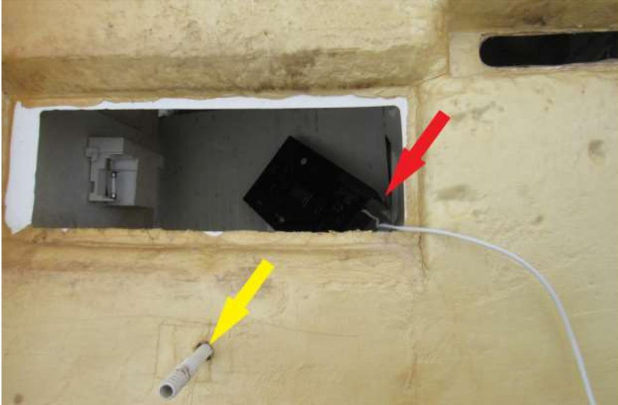
Fin fan- wire should exit the lower right corner of the foam insert (RA)
