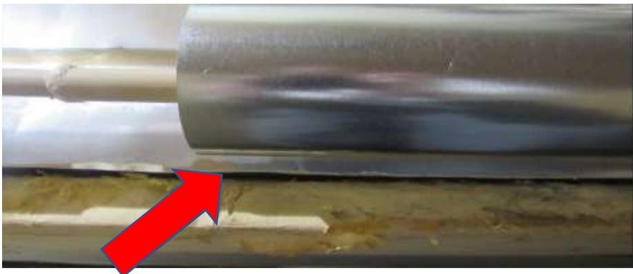
In some areas it might seem to be tight against the box, and in this area cut back enough foam on a angle to create a small gap off the unit so you can get your foam straw in to fill the void further down. **We cannot stress enough on this step because if even a small 2" gap is left open it will not cool in the fridge like it should.**
