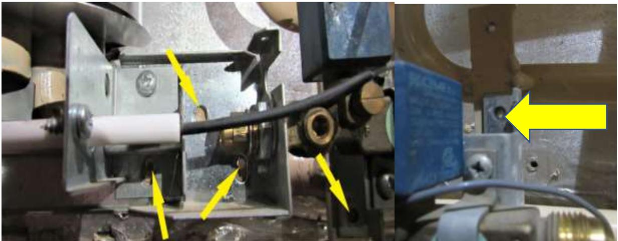
If you have the style that has a thermocouple, make sure the thermocouple is secured and is in place like it should be. When flame is lit it should be sticking into the flame at least 1/8" (RA) attach the loose ground wire anywhere to the box where its out of the way (BA)
