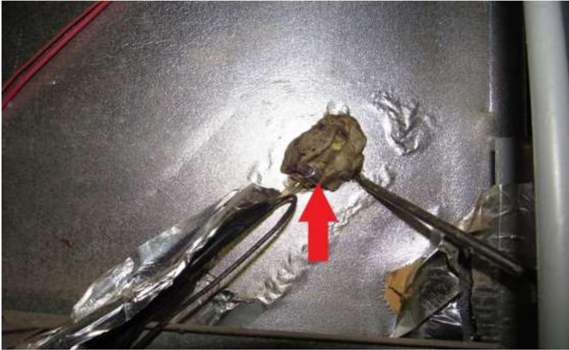
Ice maker wires need to be fed thru the unit as it is lifted up so make sure all is loose and able to slide thru (RA).
