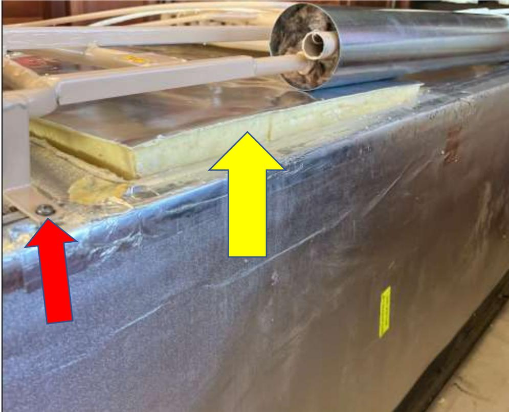
Put in bottom mounting screw in as well **(RA)**
