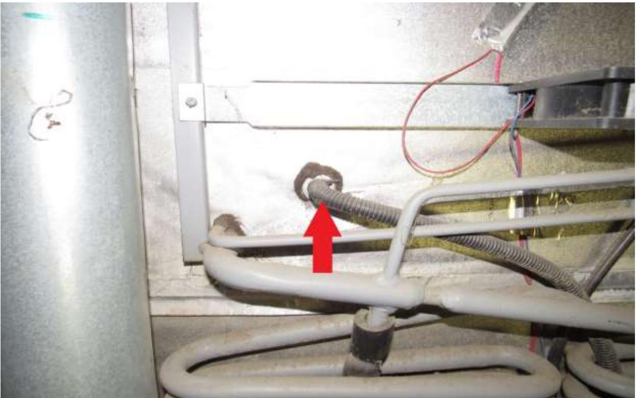
Remove wires from the fan temp switch (**RA**). Some models do not have this feature.
