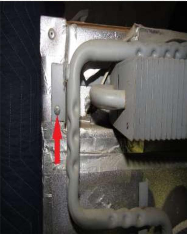
Remove water line spigot (RA) and feed water line to the bottom and swing it away from the unit.
