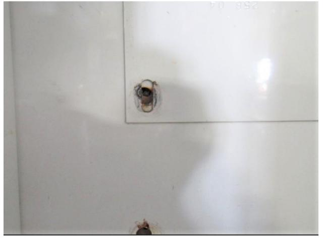
When holes are lined up, install 4 freezer screws (RA), new 2" X #10 screws provided, pull the unit tight against the back. If holes do not line up exactly you can easily angle the screw up/down side/side to get to the hole as these holes are set in approx. 1" from the front of the foam pack.
