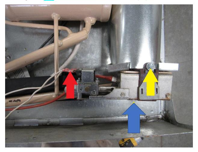
Unclip the igniter wire (RA) from the board. Also disconnect ventilation fan wires (YA).
