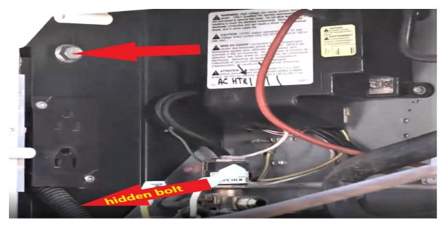
Going inside again start by removing the black trim covers on the top and bottom. Remove the two mounting screws on top and bottom (RA). Screw size and bit needed will vary from coach to coach.
