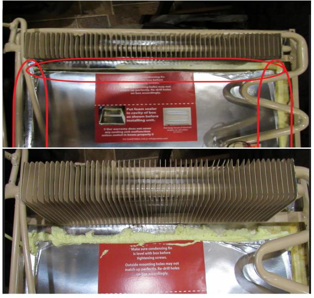
In some areas it might seem to be tight against the box, and in this area cut back enough foam on a angle to create a small gap off the unit so you can get your foam straw in to fill the void further down.
