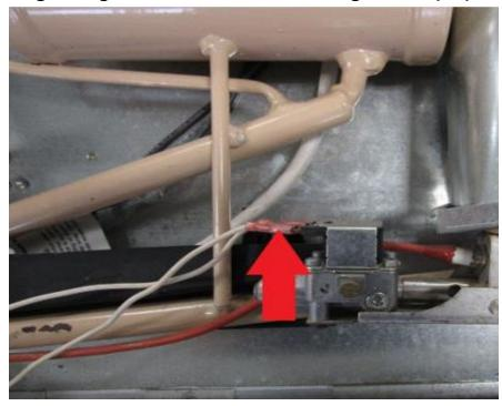
Clip the igniter wire back on the board (RA) Also reconnect ventilation fan wires (YA).
