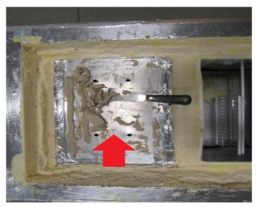
Clean off old thermal mastic from the refrigerator fin (RA).
