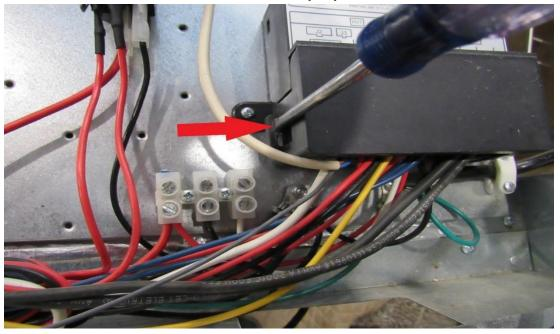
Remove igniter wire (RA) 2 black heating element wires (YA). Thermister clip(GA) do not remove any other wires from the board
