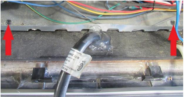
WARNING: Make sure this step is properly followed and leak checked so you don't have a gas leak.
