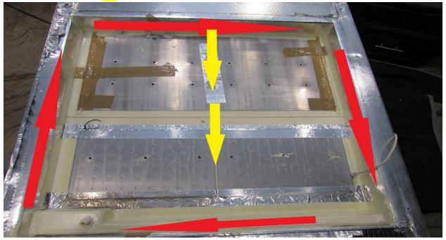
Push defrost spigot down into the refrigerator section (RA) so it doesn't break off when the new unit is set into place.
