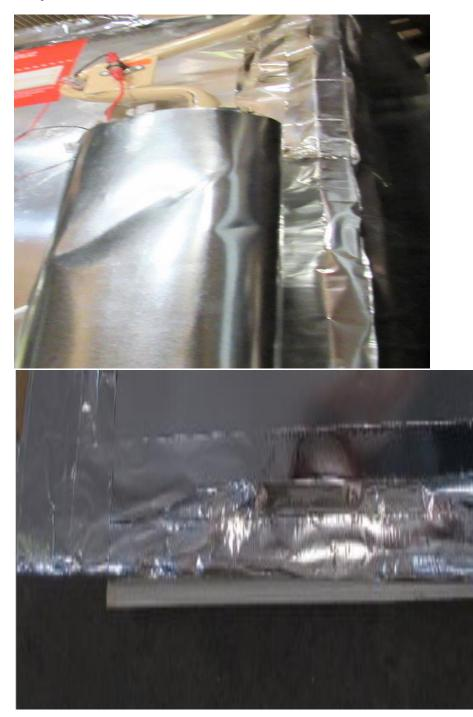
Re-install all rear mounting screws, these might not always line up perfect, do not be afraid to push or pull on the frame to get them in place (YA) if holes do not line up perfect you can use self-drilling screws to attach to the box.
