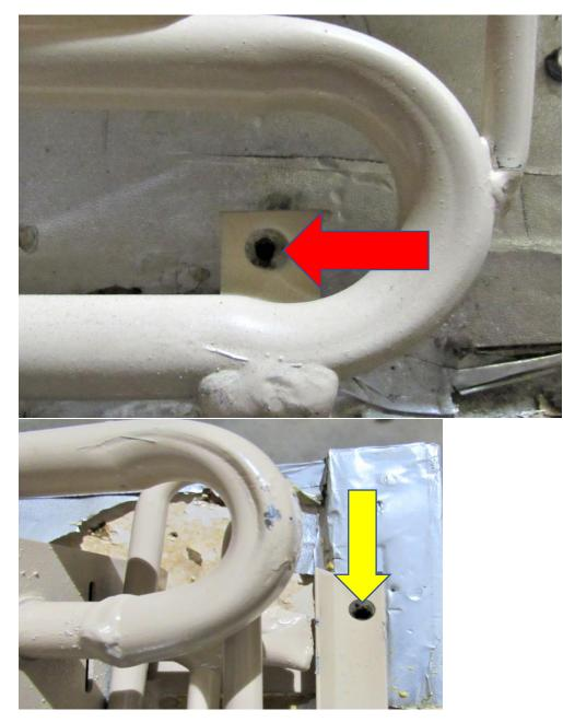
Set refrigerator upright and open the freezer doors. If holes are not aligned have the rear person lift the unit up or down or side to side till holes are aligned, or if alone you have to set fridge back down, take out mounting screws and adjust the unit to where the holes line up. It does not have to be perfect, just close enough where you can see the edge of them.
