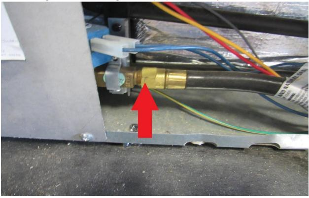
Remove LP gas hose from the gas valve (RA). Make sure your LP is turned off.
