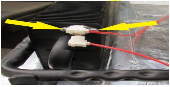
Remove the 2 screws from the fan temp switch (YA). Save them for later
