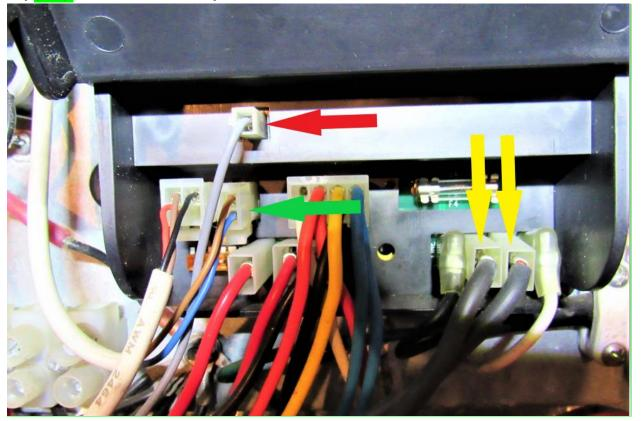
This temp sensor will have to be transferred to the new unit, carefully drill out the 2 pop rivets holding it onto the boiler stack. (RA)
