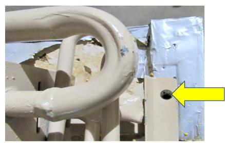
Set the unit back down on its face and remove the top mounting screw (YA).
