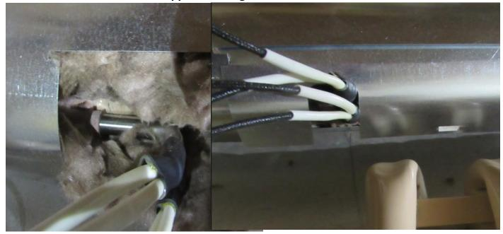
Reinstall the heat sensor, you will need 2 short screws to secure this to the boiler stack again, make sure to not boiler tube on the inside, it will just have to be attached to the thin sheet metal stack. It can be located anywhere in the red circle
