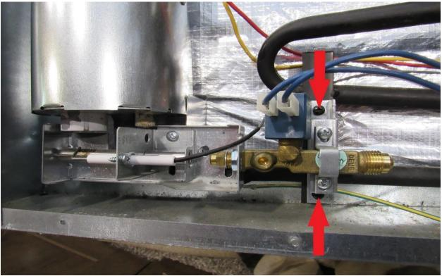
Remove the LP solenoid mounting screws (RA). Lay burner to the side
