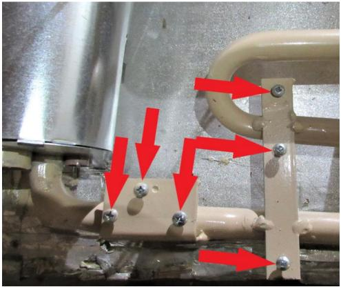
Remove these screws from burner mounting brackets (RA)
