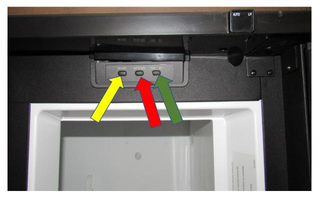
Make sure your eyebrow is now switched to "AUTO LP " the burner should now fire up and it's a good idea to recheck the gas line hook up with soap water.
