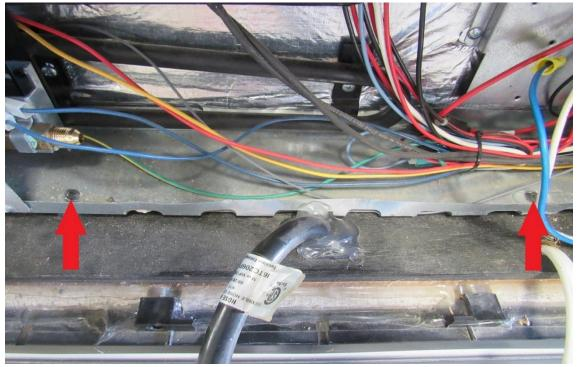
Remove the two mounting screws (RA). Location or screw size will vary
