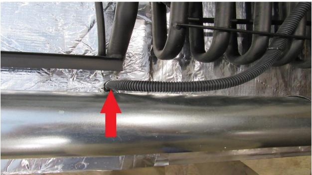
Pull out the defrost hose (RA). Set the defrost hose to the side.
