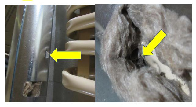
Slide the 2 heaters in these sockets making sure they are slid down as far as the heater lets them be slid, now tuck the insulation around the heaters and boiler tube and secure the heater flapper cover again.
