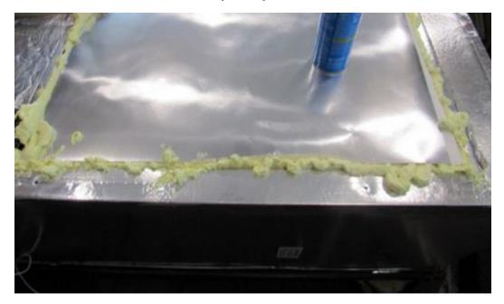
After filling all gaps with foam, follow up with covering the edges with the supplied aluminum tape. This does not serve as a seal but for cosmetic purposes only.
