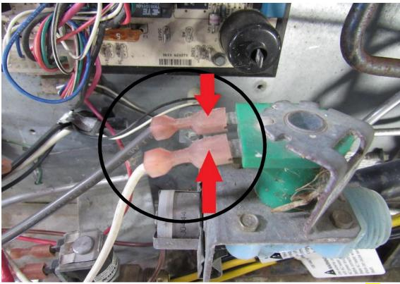
Remove the ice maker solenoid brown and white wires (RA).
