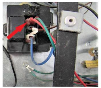
If the recall device is to be taken out, remove the blue wire (YA). Loop red wire as shown creating a "jumper" (RA). The 2 spades "limit in & limit out" should be looped together as seen (RA)
