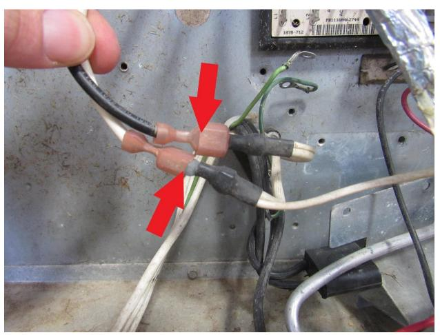
Disconnect the 120V ice maker wires, mark these to make sure you know which ones they are later, because these can be confused with the 12V fan wires (RA).
