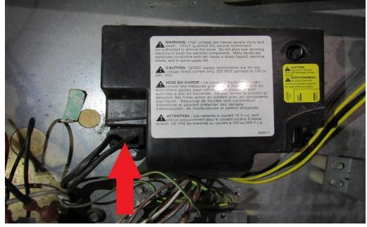
Plug the igniter into the board (RA) as shown.
