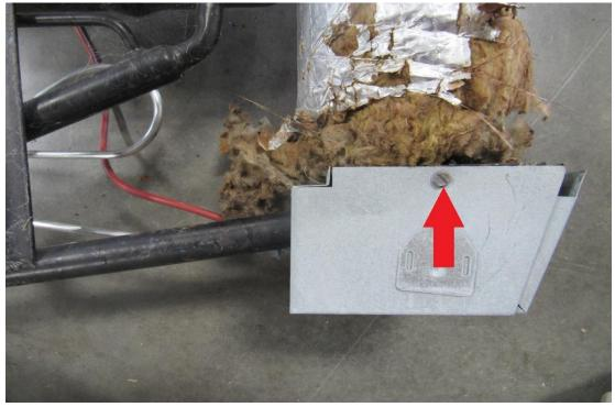
Remove the ¼" screws (RA) and set the burner housing to the side.
