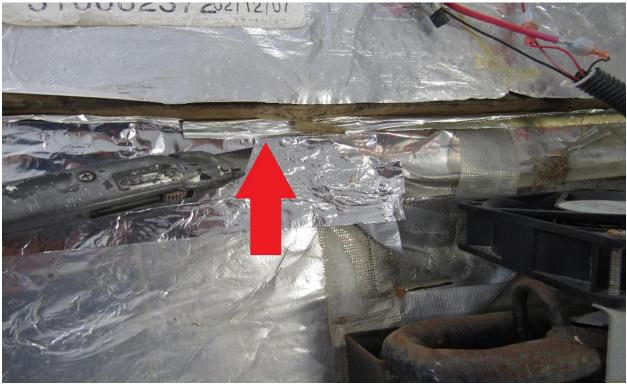
If old unit is taped along the sides, cut tape with knife (RA).
