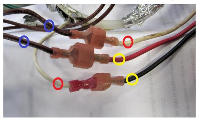
These 6 wires need to interconnect, wires are color coded to previous pics.
