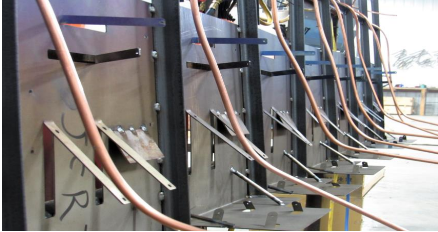
Units prepped for compressors
